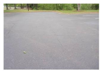
to include, including tree root damage, cracks, depressions, and potholes which could pose trip hazards.
